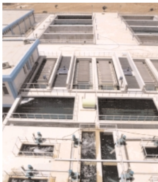
Flocculation, sedimentation and filtration tanks
