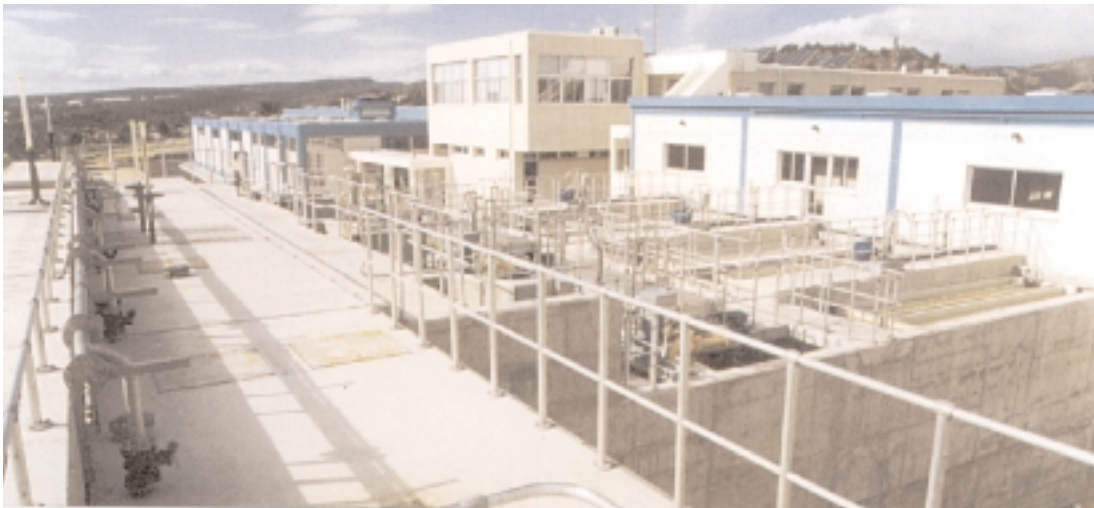
General view of Limassol Water Treatment Plant
