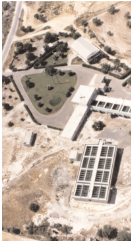
Aerial photograph of Khirokitia Water Treatment Plant
